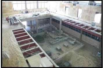
**Figure 2:** By 2009 the foundations for Ranefer's house were being laid down. The square pillars are where the four columns of the front reception hall will stand.
