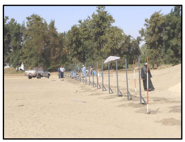
**Figure 4:** Iron Fence posts ready for fencing along the survey line.
